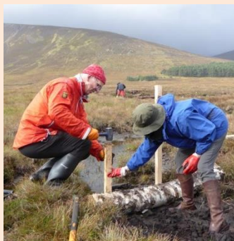
NE Scotland Members group peatland restoration by dam building on Glen Muick, Balmoral estate
