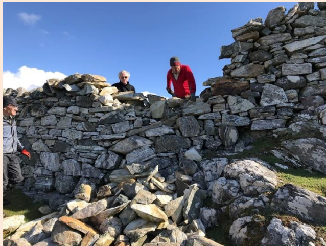
Above repairing drystone dyking on Isle Scalpay below a dyke fully repaired at Glenridding
