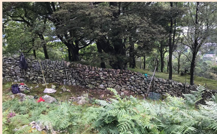
Above repairing drystone dyking on Isle Scalpay below a dyke fully repaired at Glenridding
