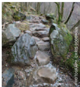
Digging deep: a Lochinver-based contractor working at Sandwood recently (left); sensitive path repairs incorporating existing rock features at Steall Gorge, Nevis (below)
