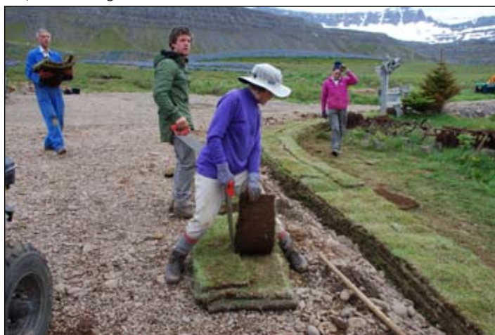
Turf wall building at Skalanes
