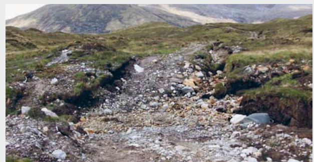
A hill track showing erosion, leading to silt run-off, in and around a stream
